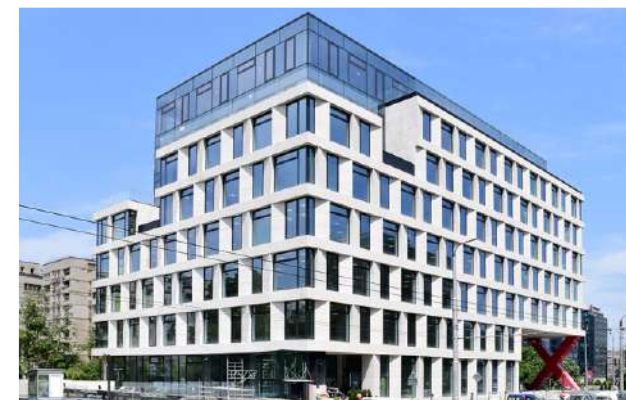
Project: GRAFIX Location: Sofia, Bulgaria Architect: LP Arch Ltd. Contractor: GP Group Sofia AD Year: 2018
