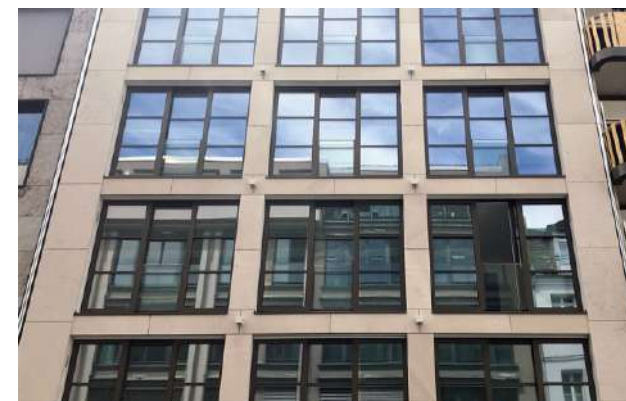
Project: LINIENSTRASSE Location: Berlin, Germany Architect: Dr. Krause Architekturbüro Contractor: WETRI GmbH Year: 2018
